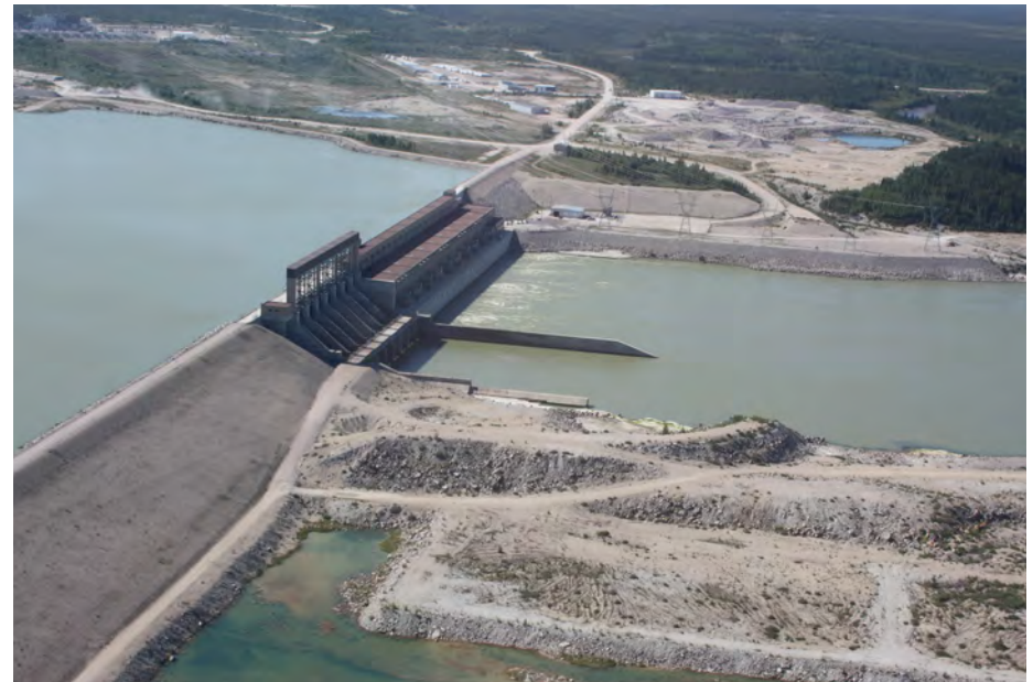
Limestone Generating Station
