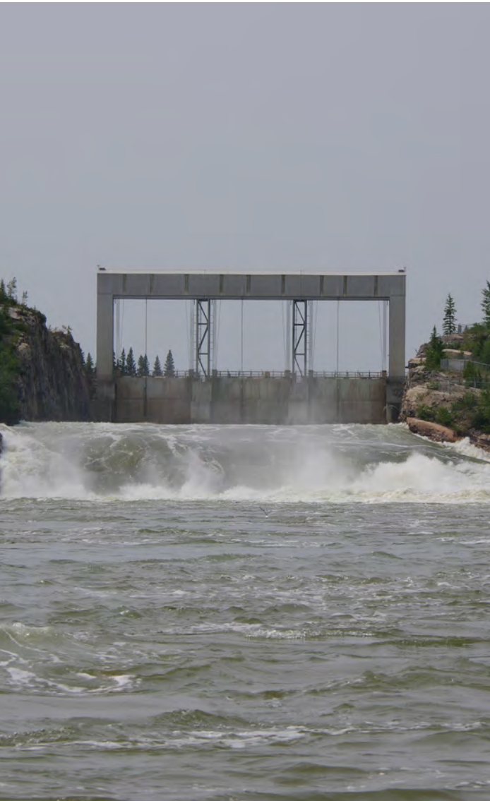
Notigi Control Structure
