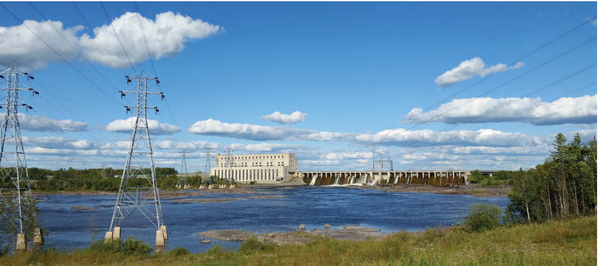
Seven Sisters Generating Station
