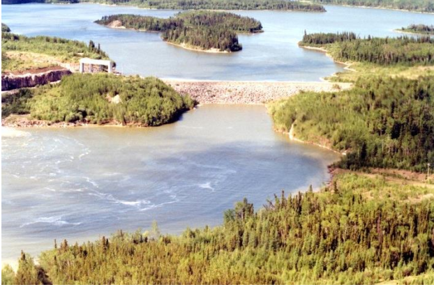
Notigi Control Structure.
