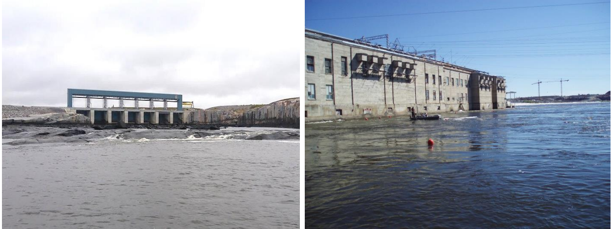
Pointe du Bois GS and spillway.
