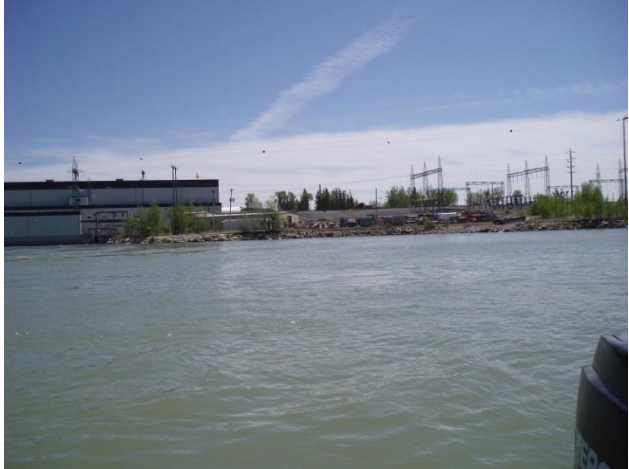
Jenpeg Generating Station.
