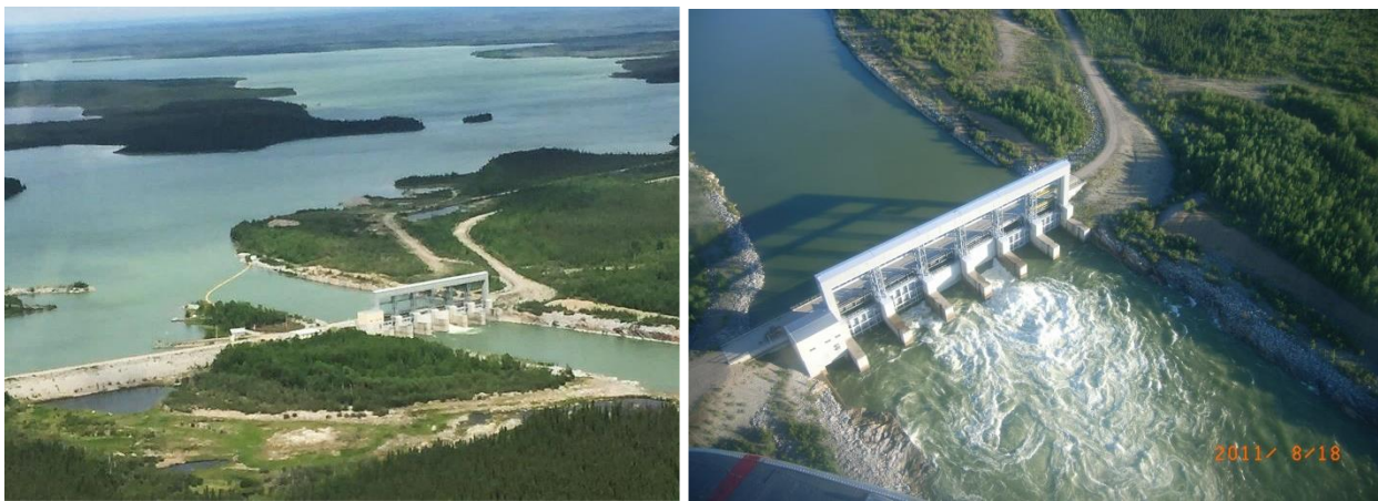
Missi Falls Control Structure at Southern Indian Lake.
