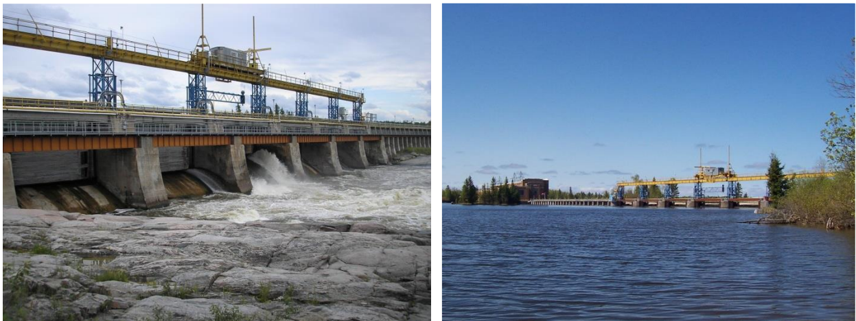
Slave Falls GS and spillway.
