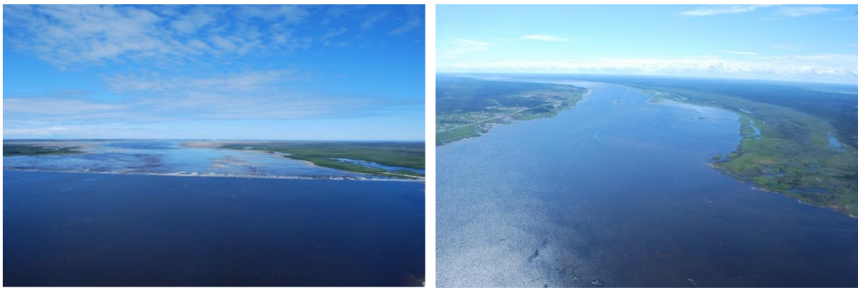
Lower Churchill River at the Churchill Weir.
